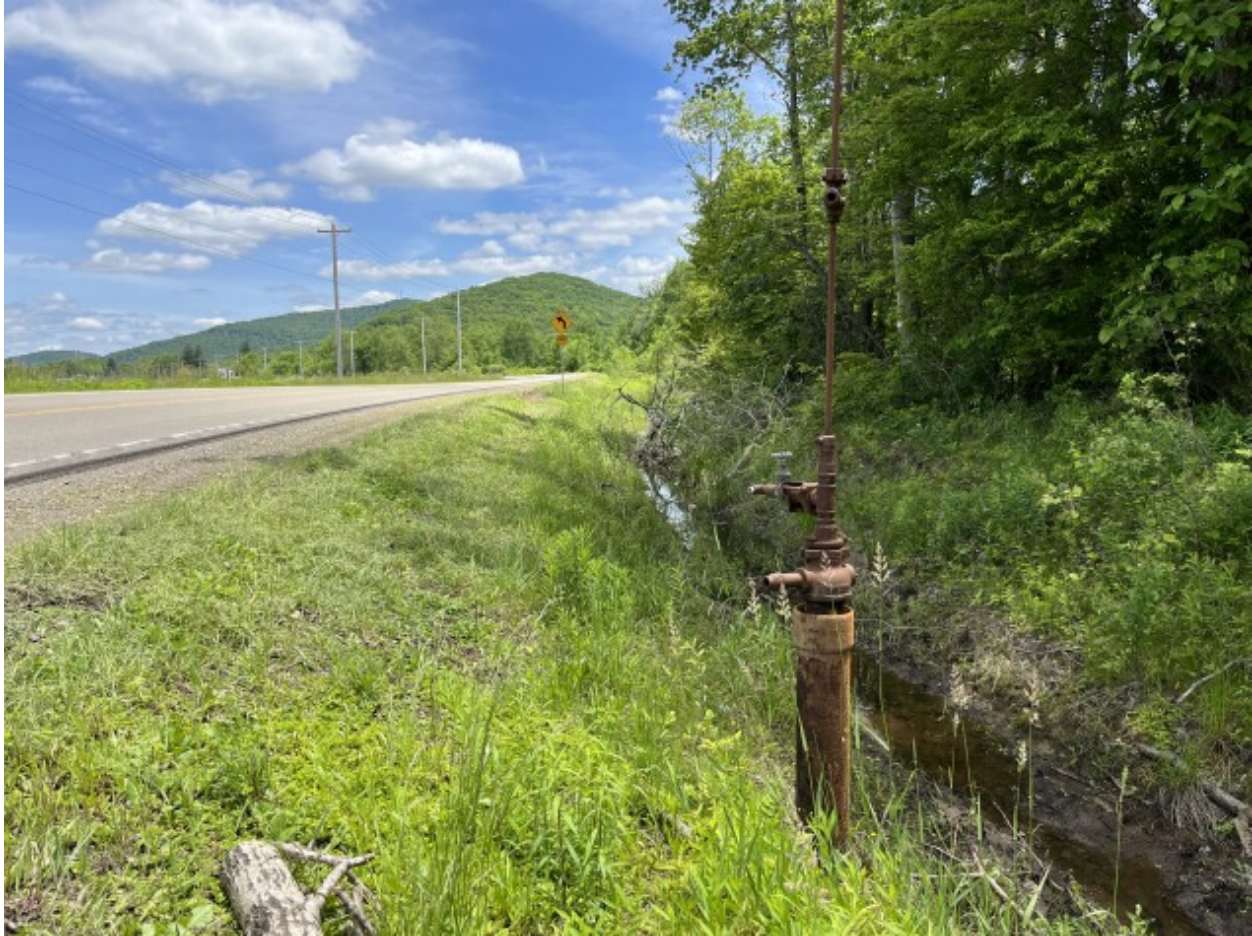
An abandoned oil well on the side of a highway in Cattaraugus County, N.Y.
